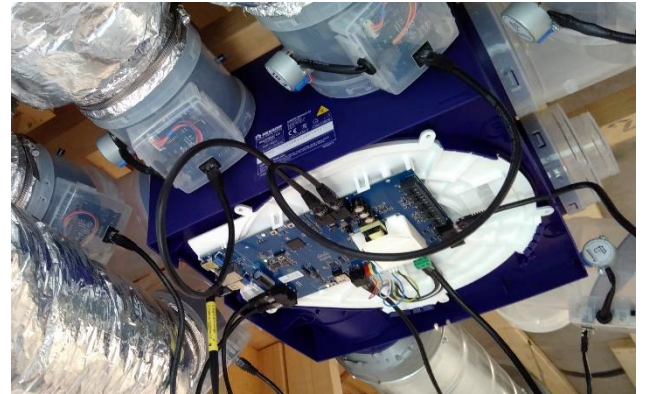
Figure 7.4 Renson Healthbox air handling unit, with cover removed for access to connections
